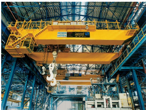
160/60/30 t x 22m (esfarayen steel co)
